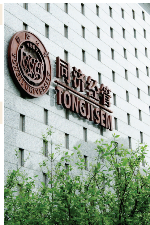
Tongji Building A
