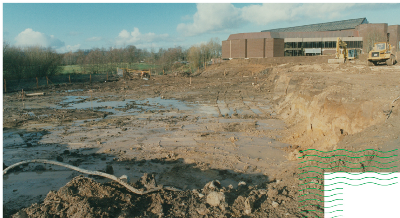
Laying foundations of the Glucksman Library
