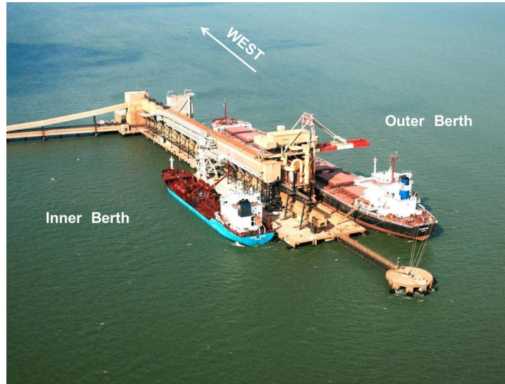
Figure 1: Rusal Aughinish’s jetty.
