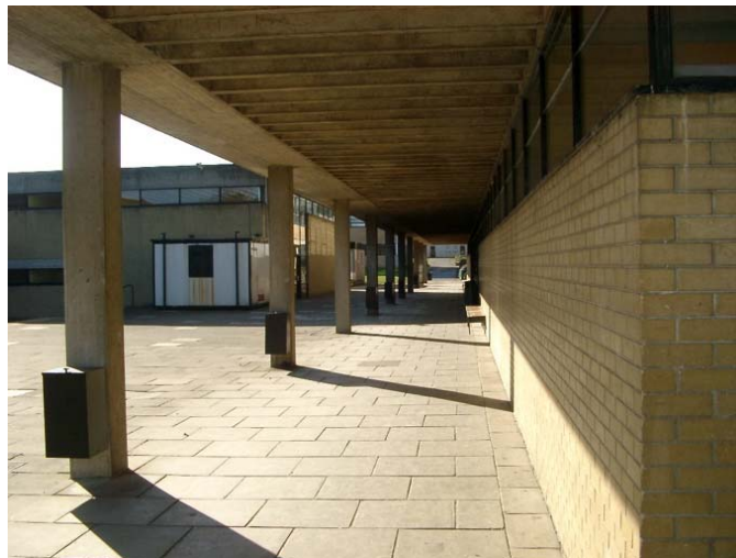
Sunlight on the Classroom Block
