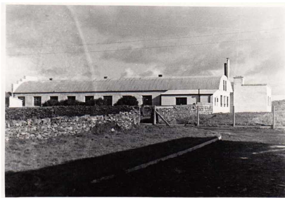
[below] The factory premises of Dalcash Labels Ltd. seen from the Hill House.
