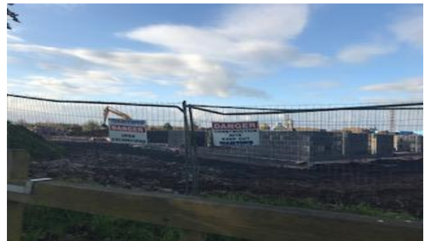
Building of the respite centre in progress
