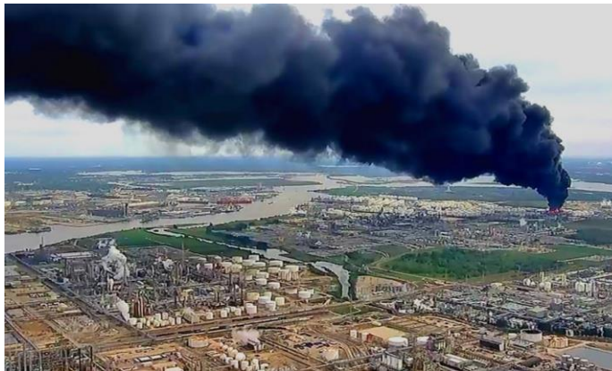
Figure 1: Plume of black smoke rising from ITC's tank farm fire. Image source: U.S. CSB
