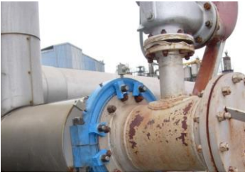
Figure 1: A leak-sealing clamp (blue) fitted to a flange. Image not related to this incident. Image source: https://leaksealing.com/
